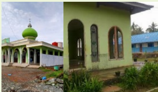
Renovasi masjid / Mosque renovation
