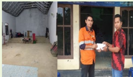
Renovasi gereja / Church renovation
