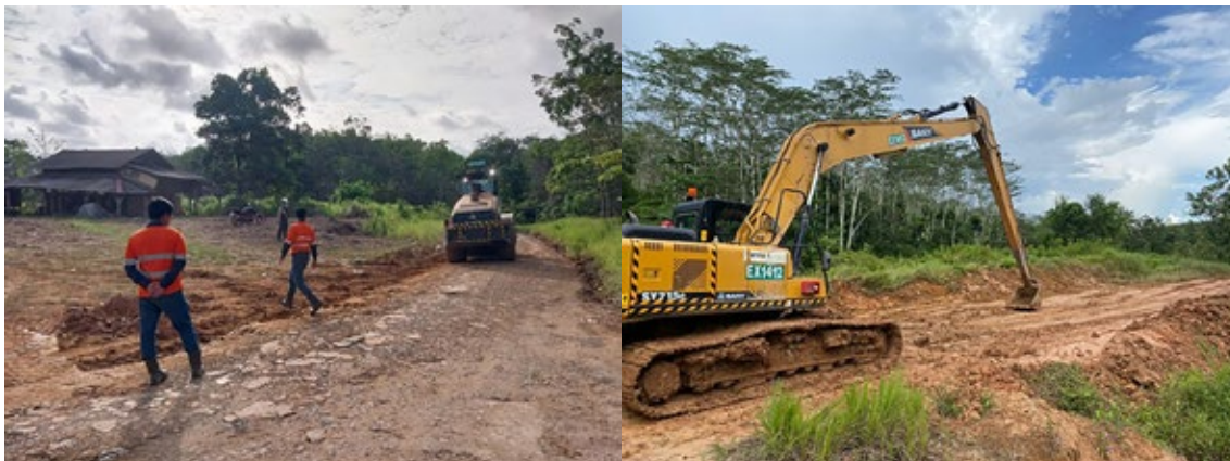
PT Darma Henwa Site Kintap Coal Project melakukan kegiatan perbaikan jalan warga di RT 10 Desa Sumber Jaya PT Darma Henwa Site Kintap Coal Project carries out road repair activities for residents in RT 10 Sumber Jaya Village
