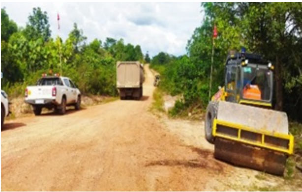
Penimbunan dan perbaikan jalan desa tebangan lembak KM10 Backfilling and repairing KM10 tebangan lembak village road
