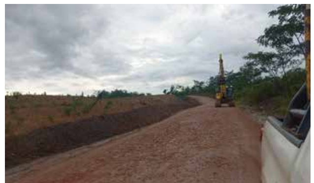
Perbaikan akses jalan Desa Segading yang terputus akibat tergerus luapan air Repair of Segading Village road access that was cut off due to overflowing water
